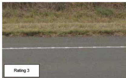
Rating 3 Slight obstruction to either runoff entering the table drain or along the table drain invert through scour, siltation or vegetation build up typically in the range of 30 to 50 mm.
