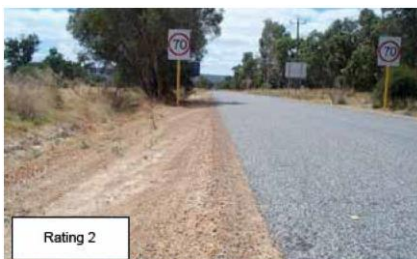
Rating 2 May be some obstruction in the form of vegetation build up or scour or siltation. This is less than 30 mm.
