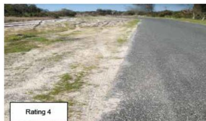
Rating 4 Moderate restriction to drainage flow across the shoulder. Scouring present with depth between 40 and 80 mm. Soft patches of unconsolidated material over between 10 and 50 % of the area.
