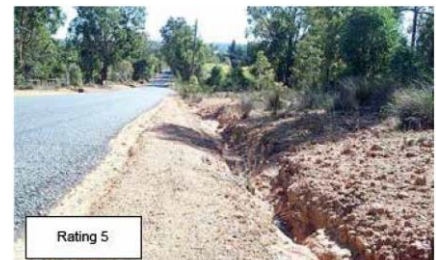
Rating 5 Major restriction to drainage flow across the shoulder. Scouring present greater than 80 mm deep.
