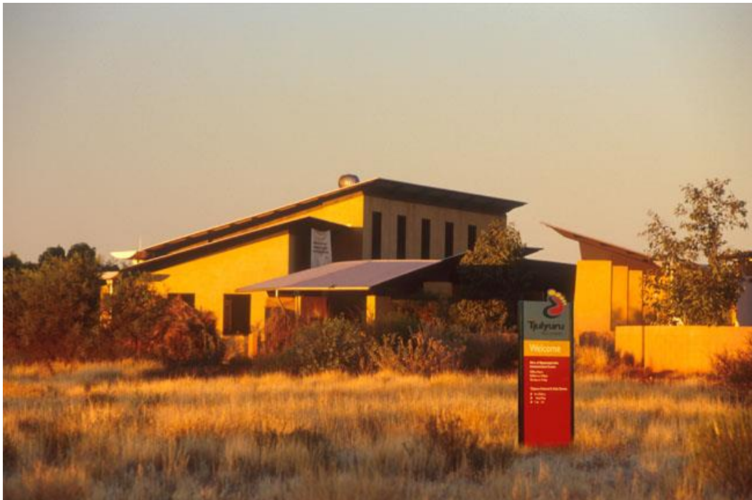
Shire of Ngaanyatjarraku Offices, Tjulyuru Cultural and Civic Centre, Warburton
